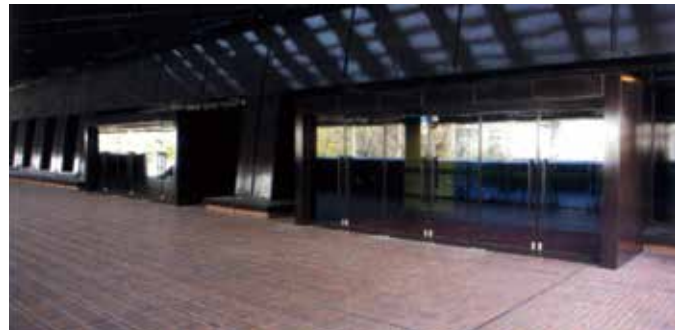
2階入口 Entrance 2nd floor
